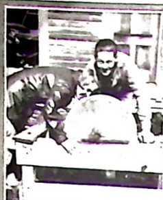
Here is the Grindstone, Janice.
