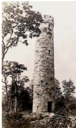
Tower without any cab - original construction (Courtesy of Shelburne Historical Society)
